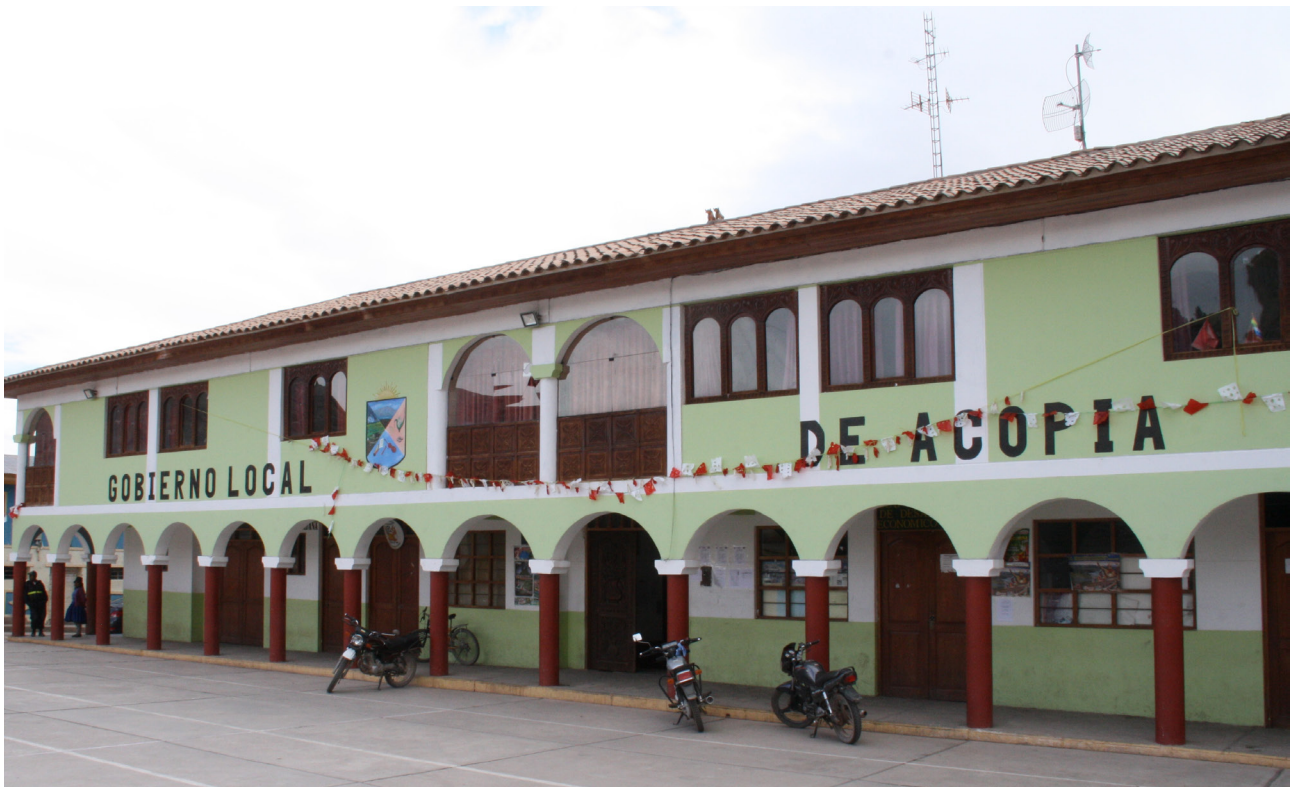
Façade of the Town hall in the District of Acopía (Zabalketa)
